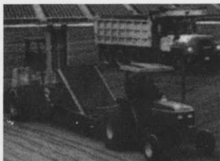
Stripped and installed Jacobs Field Cleveland Indians
