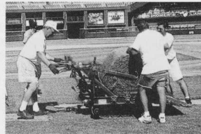
ST. LOUIS CARDINALS STRIPPED & INSTALLED 42"
