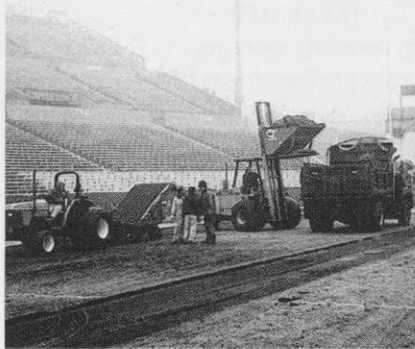
NEW ENGLAND PATRIOTS STRIPPED FIELD INSTALLED 2" THICK 48" ROLLS
