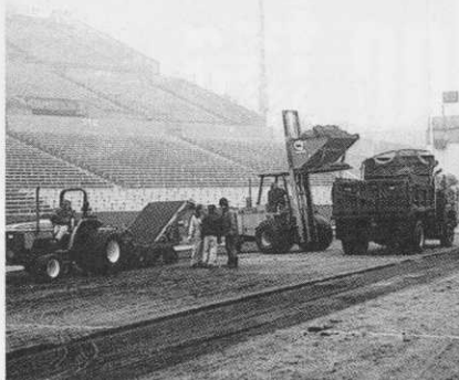
NEW ENGLAND PATRIOTS STRIPPED FIELD INSTALLED 2" THICK 48" ROLLS
