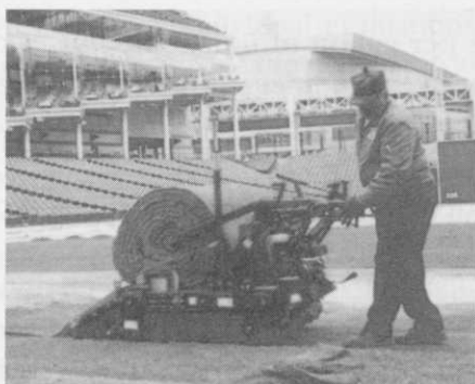
INSTALLED CLEVELAND INDIANS IN 42" AND 48" ROLLS
