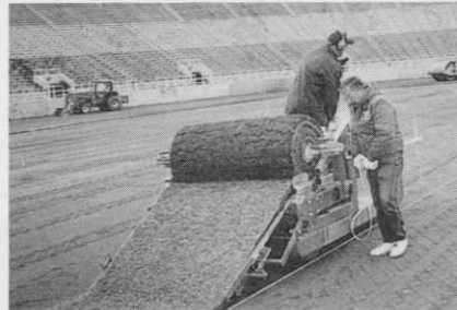
INSTALLED OHIO STATE (AND STRIPPED) 2" THICK TURF 48" ROLLS
