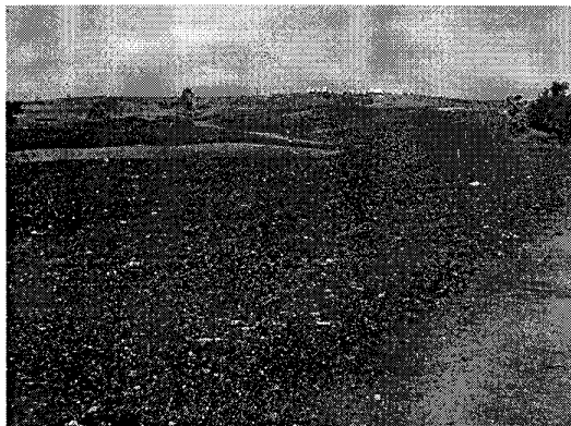
Fig. 3. Topsoil cap in place on fairway #10.
