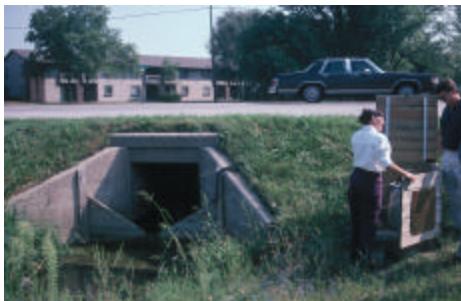
Storm water from a residential area is monitored as it enters the Kampen Golf Course at Purdue University.
