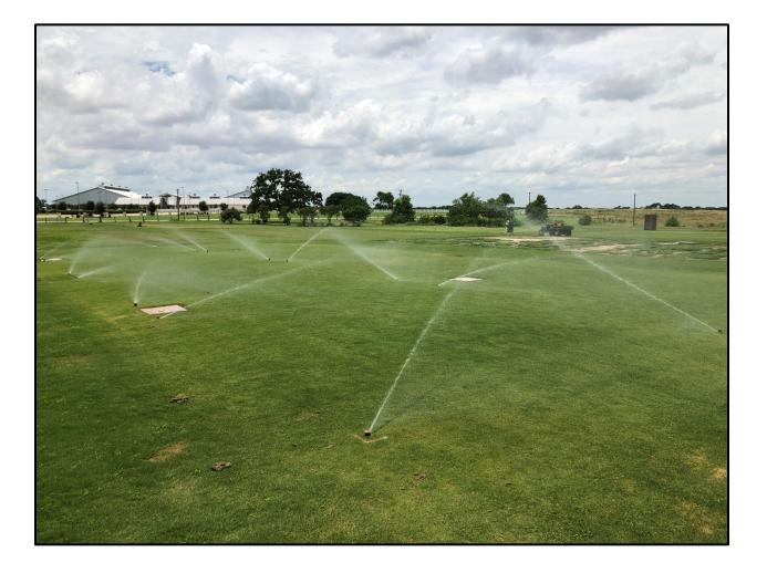
**Figure 5**. Image of the sand-capping irrigation facility at Texas A&M University, College Station, TX. The facility contains 16 independently irrigated zones and was established in 2018 with 'Latitude 36' hybrid bermudagrass atop a 7" sand-cap.
