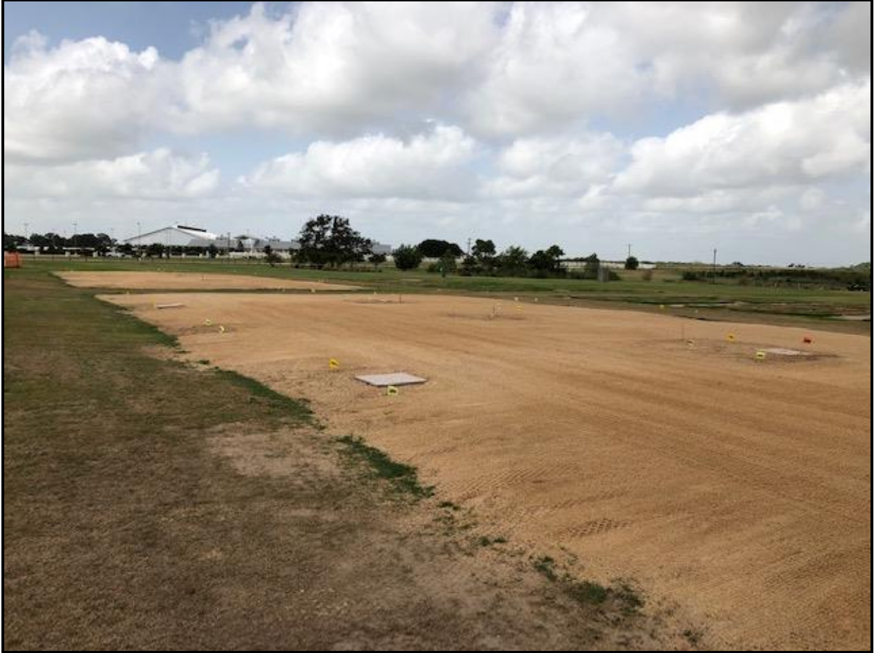
Figure 3. Image of the sand-cap final grade prior to sprig establishment in early August 2018.
