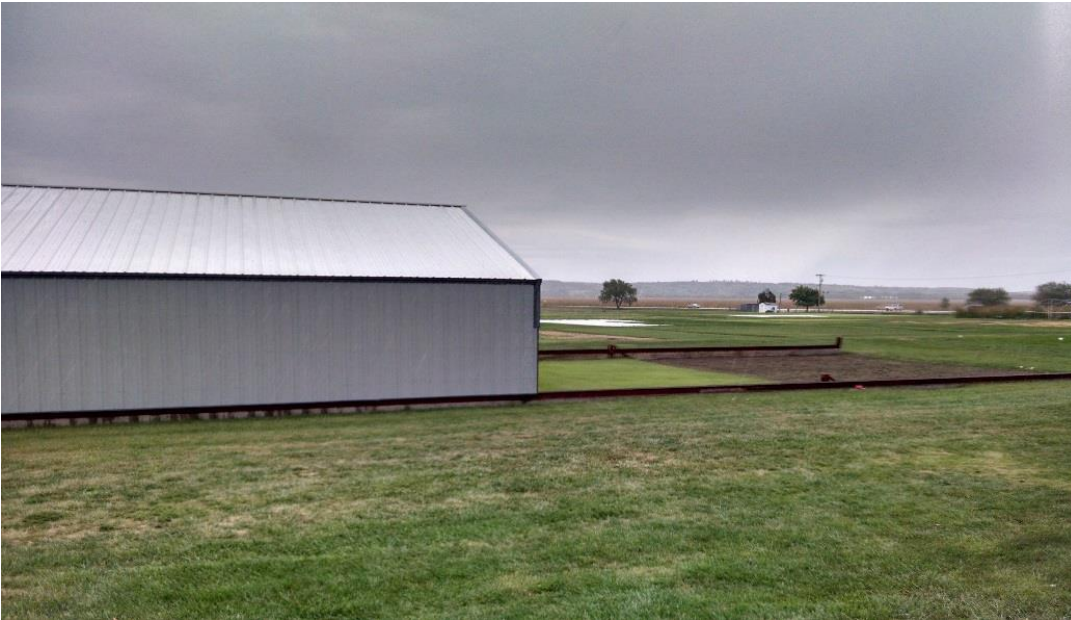
Figure 1. Automated rainout shelter moving across plots activated by 0.01 inch of rain.
