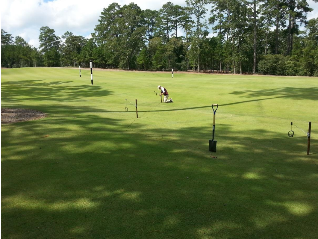
Figure 7. Mounted PAR sensors being installed in a Zeon zoysiagrass fairway at Bluejack National Golf Club, Montgomery TX for determination of minimal DLI needed to achieve acceptable turf quality. Five PAR sensors were mounted at varying distances into the fairway from the pine tree shade line at the south edge of the fairway during late September and early October 2017.
