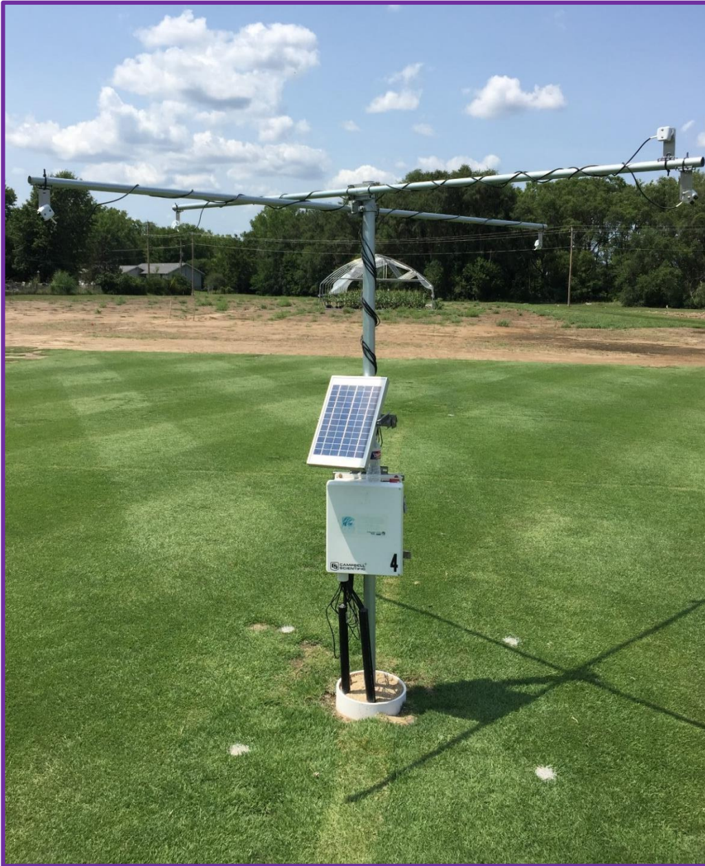
Figure 4. Initial site setup.
