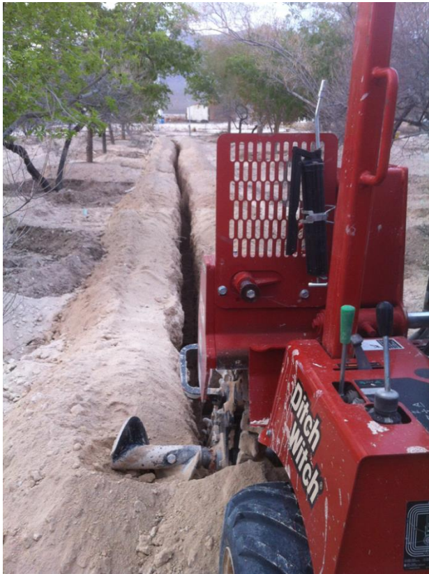
Trench dug to 120 cm to cut roots, isolating each tree
