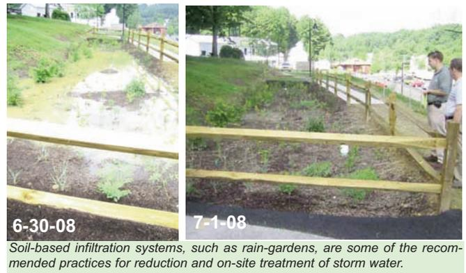
Soil-based infiltration systems, such as rain-gardens, are some of the recommended practices for reduction and on-site treatment of storm water.
