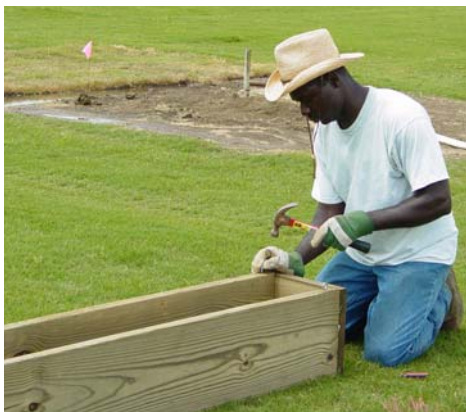
Construction of runoff plots allows researchers to compare different pesticides in their abilities to be washed off both bermudagrass and zoysiagrass by simulated rainfall at MSU.
