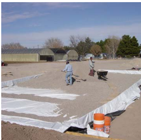
Irrigation research plots were built to study the impact of irrigation type (sprinkler vs. subsurface drip irrigation vs. subirrigation) and type of rootzone mix (straight sand vs. sand mixed with peat vs. sand mixed with urea-formaldehyde polymer) on irrigation efficiency and turfgrass performance of 'Bengal' creeping bentgrass.
