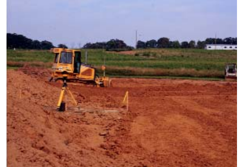
In mid-July, the area was re-graded to create three small (12 ft by 30 ft), and large (40 ft by 125 ft) size plots, each having a uniform 3.5 % grade with no measurable cross-slope.
