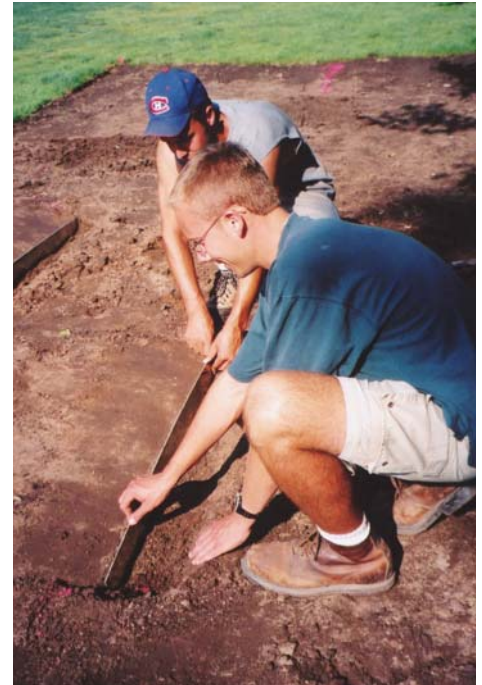
Galvanized steel runoff collection flumes (1 m) were installed during August.
