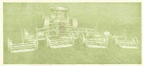
The Worthington Convertible "Multigang" gang mower having seven units arranged in two rows, cutting a swath of sixteen feet. In combination with the Worthington tractor, this wonderful apparatus will cut an acre of grass in four minutes. Its patented hinged frame permits it to be changed or converted immediately into a five-unit gang; a three-unit one, or into a single-unit Sulky, as occasion may demand.
