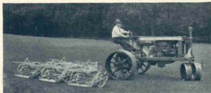
The square-turn feature of the Fairway enables it to cut close to trees and shrubs.
