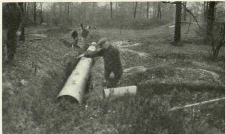
INSTALLING ARMCO PIPE AT THE CLEVELAND COUNTRY CLUB Photo shows Bert G. Sheldin, greenkeeper, helping lay a 30-inch pipe on No. 5 fairway. A minimum amount of excavation, quick placing and easy aligning are characteristics which speeded up the work
