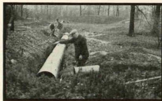
Bert Sheldon, greenkeeper at the Cleveland Country Club, superintending installation of Armco Perforated Pipe on his course
