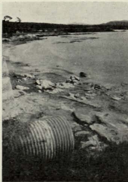
ARMCO AT PEBBLE BEACH Showing how an open ditch across No. 18 fairway was completely enclosed in an Armco Corrugated Iron Pipe
