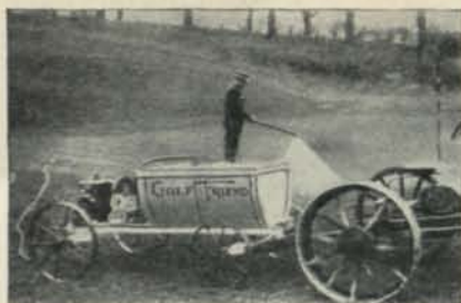
One of the smaller sprayers at work, driving a fine spray into sod of putting green with special Golf Gun.
