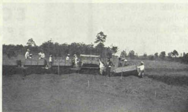
BUILDING NO. 18 GREEN AT THE TOKIO COUNTRY CLUB The Japanese do most of their work by hand labor and at one time Mr. Penglase had 600 men working on the construction of this course. The details as he describes them are extremely interesting.
