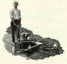
inally, a 24-inch swath mower. A great feature of the attachment is that it can be raised while mower is moved from place to place.
