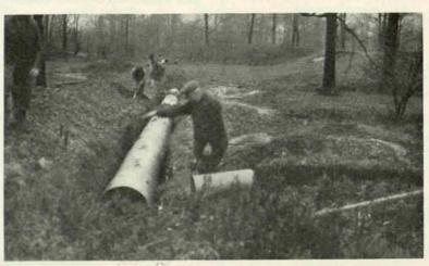
INSTALLING ARMCO PIPE AT THE CLEVELAND COUNTRY CLUB the smaller streams under the fair- Photo shows Bert G. Sheldin, greenkeeper, helping lay a 30-inch pipe on ways in tile of a capacity sufficient No. 5 fairway. A minimum amount of excavation, quick placing and easy aligning are characteristics which speeded up the work
