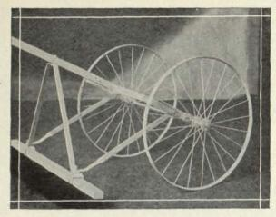
This is a valuable machine, for the greenkeeper, having various uses, some of these are, rubbing in compost after top-dressing, brushing worm casts, bringing the runners of bent to the surface where they can be cut, brushing the greens in the early morning, getting the dew off, and giving the grass a chance to dry off, so that the greens can be cut sooner, also "lessening the danger of Brown Patch."
