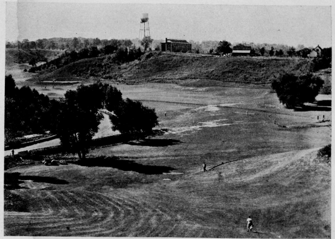
Holes Numbers Eleven and Thirteen in the hills and valleys of the course at Durand-Eastman Park, Rochester, New York.
