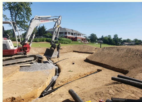
Right side #18 green pipe and gravel installation
