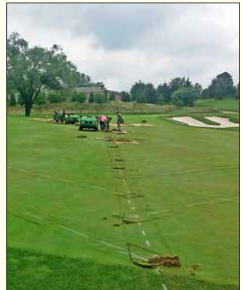
Mike's team completing drainage work at Riverbend
