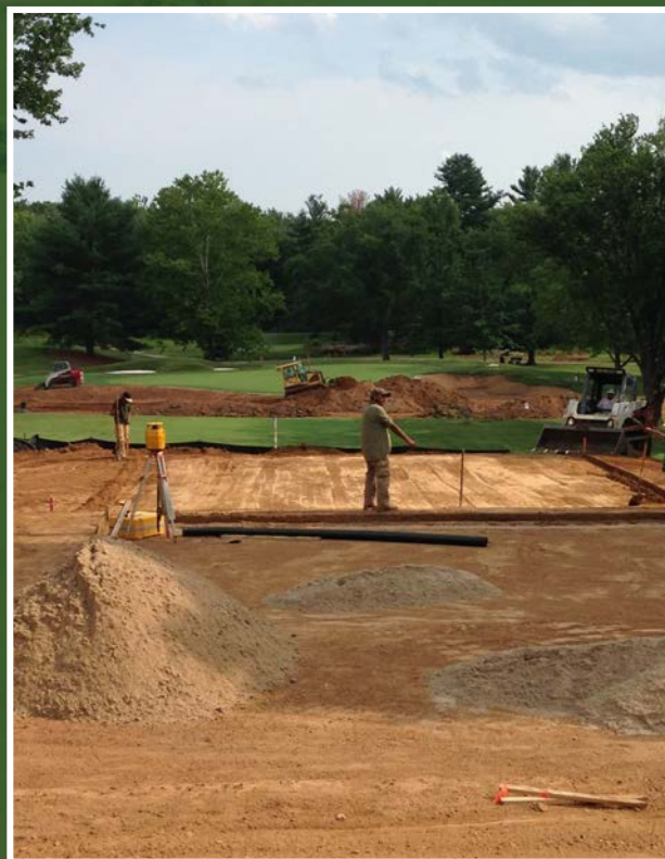
Above: Hole 14 During Construction
