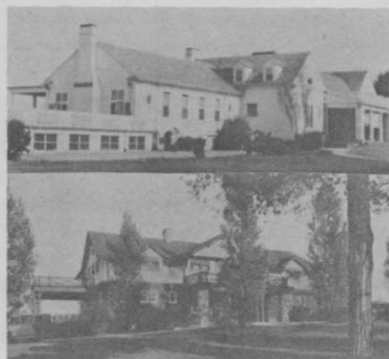
Top, the second WG&CC clubhouse that was torn down in 1958 to make way for the present one; bottom, the original Glebe Road clubhouse that burned to the ground in 1936.
