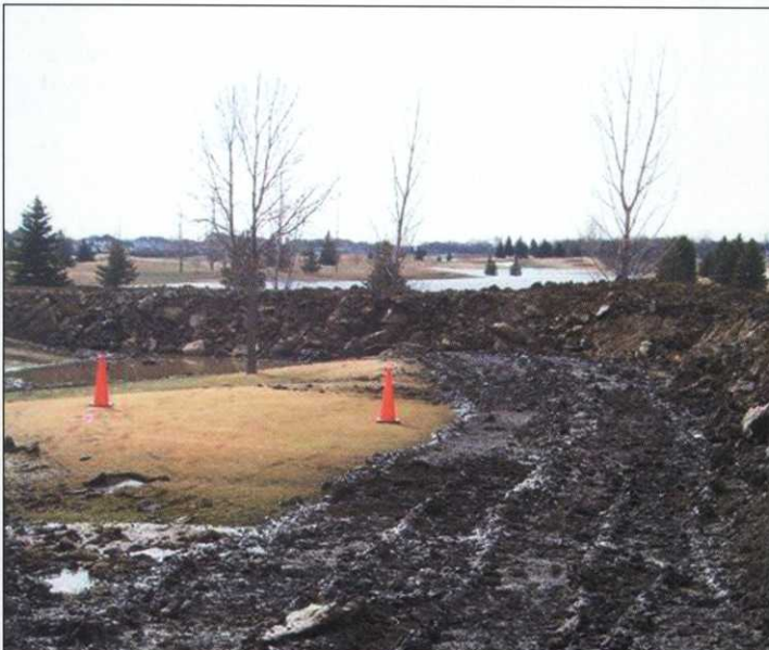
Dikes were formed to protect parts of the course and neighboring houses.
