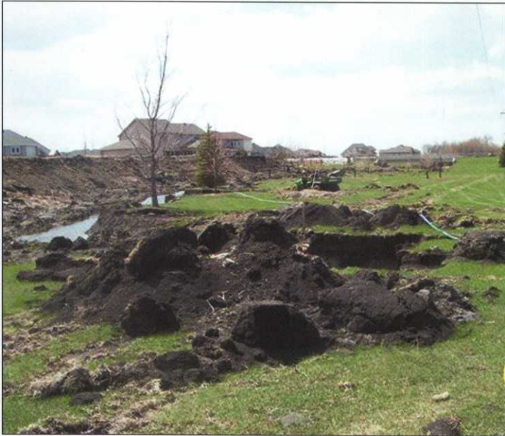
Pumping holes to check for damage to utilities.
