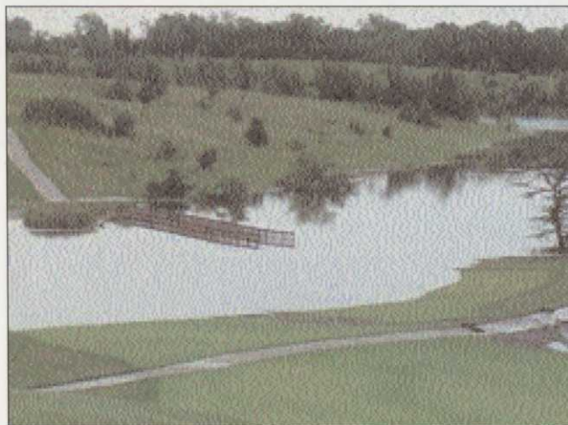
Photos of "The Preserve at Honey Creek" project designed by Herfort Norby Golf Architects for the Iowa Dep't of Natural Resources about an hour west of Des Moines. These bridges were originally set about 10' above the creek bottom. Water has now risen over the railings. The course was scheduled to open the first week of August but it didn't happen. - Kevin Norby
