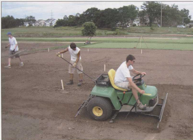
Ben Pease's horticulture crew building a raised soil green to be used for bentgrass variety trials in Madison, Wisconsin. - Ben Pease
