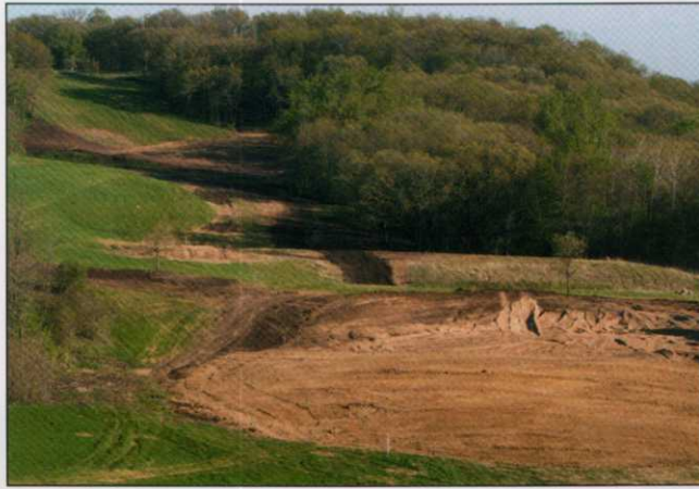
Rough grading of first and second hole at Fort Ridgely.
