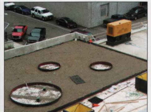
9. Installation of finishing sand layer.
