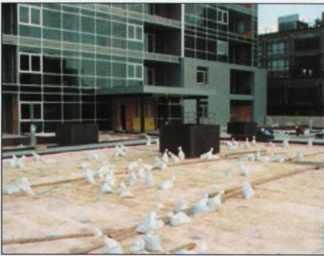
1. Roof membrane and insulation.
