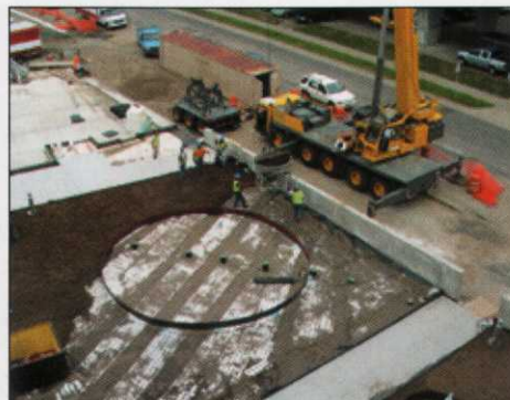
8. Installation of Netlon mesh layer.
