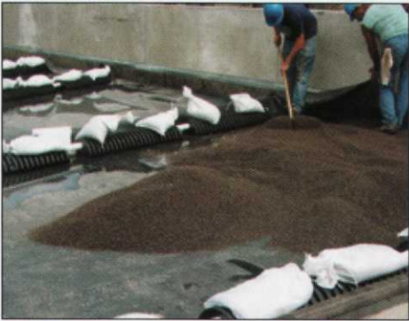
4. Installation of light weight rock.
