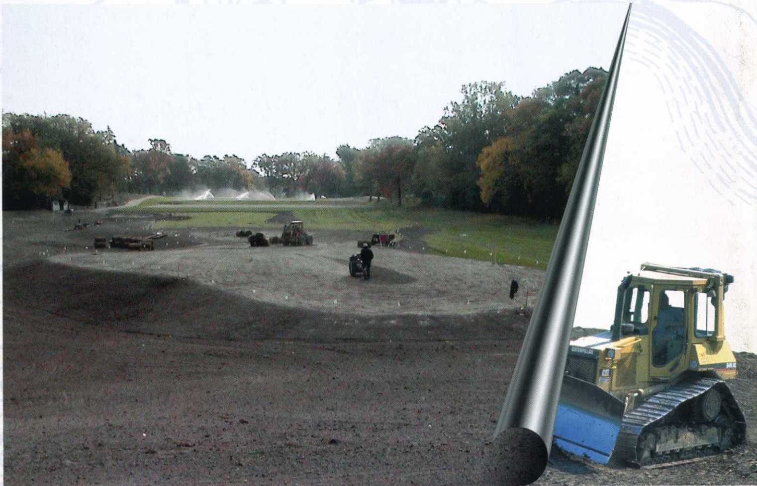
Interlachen Country Club - Driving Range Improvement Project
