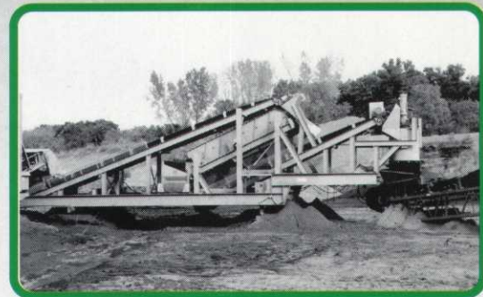
Screen deck and stacking conveyor.
