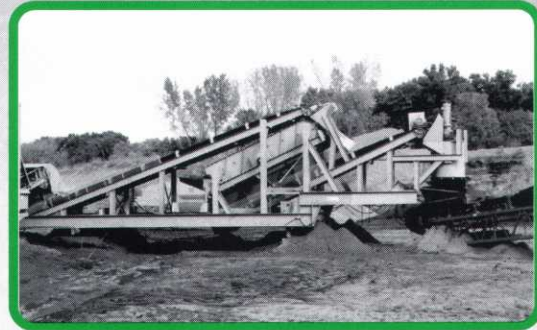
Screen deck and stacking conveyor.
