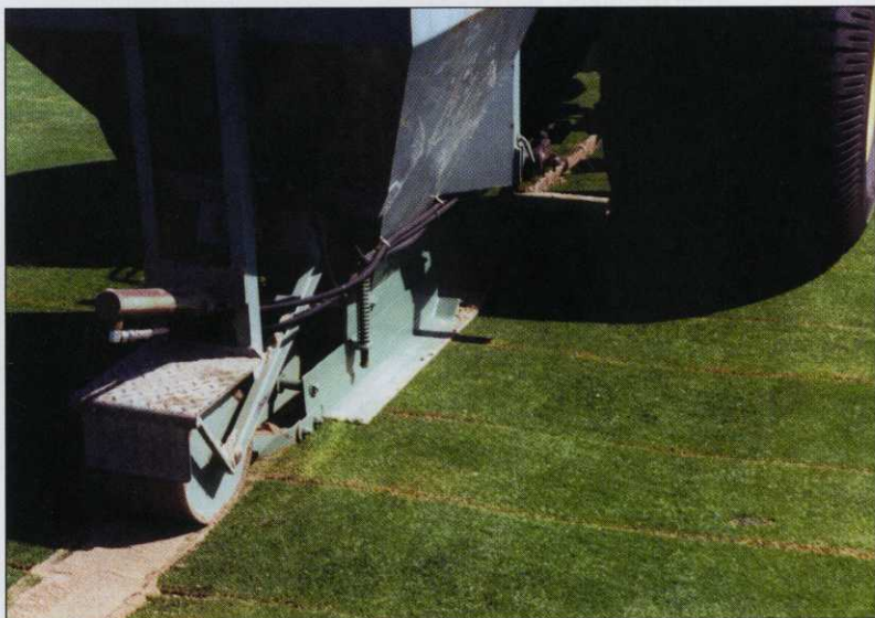
The final stage is backfilling with sand and compacting.
