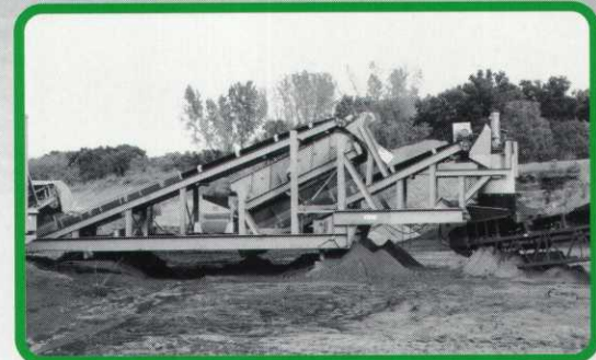
Screen deck and stacking conveyor.
