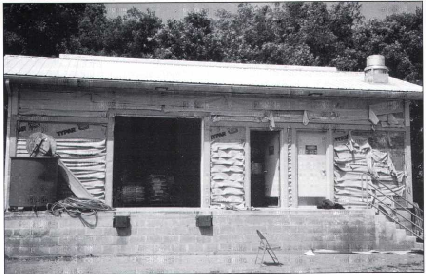
THE CHEMICAL BUILDING AT THE CHASKA TOWN COURSE was spared of any interior damage but the radiant heat from the maintenance building fire caused some exterior damage.
