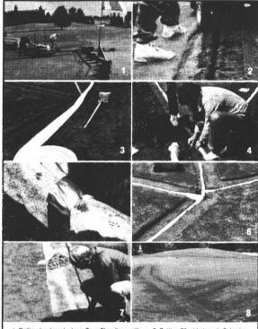
Rolling back sod where TerraFlow lines will run. 2. Cutting 2" wide trench. 3. Laying TerraFlow lines in 12" deep trench. 4, 5. Joining TerraFlow lines using only a utility knife and duct tape. 6. Fully installed TerraFlow System. Workers backfill with site soil, puddle with sand. 7. Replacing sod. 8. Completed TerraFlow System. Installation time: about 100 ft. per hour. (Photos by Greg Fast, Turf Irrigation Supply, Englewood, Colorado.)
