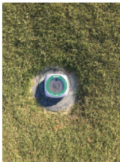
Sprinkler level check
