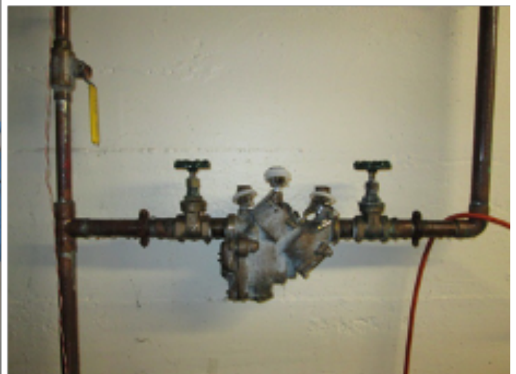
Above: Reduced Pressure Principle or Reduced Pressure Zone Device (RPP or RPZ): Once installed, this device must be tagged and inspected by a licensed plumber. An RPZ is made up of two independent check valves with an automatic pressure differential valve located between the two valves. If either check valve leaks, the relief valve will discharge to the atmosphere. If located properly, this device could be used by itself for prevention of backflow when filling application equipment and/or rinsing or washing empty pesticide containers and application equipment.
