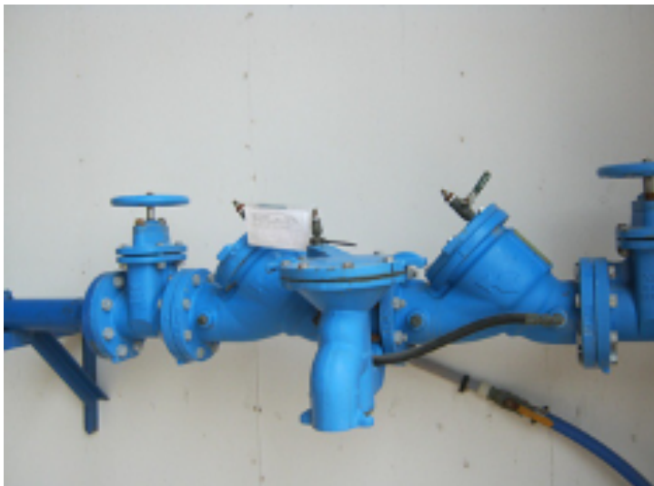
Above: Reduced Pressure Principle or Reduced Pressure Zone Device (RPP or RPZ): Once installed, this device must be tagged and inspected by a licensed plumber. An RPZ is made up of two independent check valves with an automatic pressure differential valve located between the two valves. If either check valve leaks, the relief valve will discharge to the atmosphere. If located properly, this device could be used by itself for prevention of backflow when filling application equipment and/or rinsing or washing empty pesticide containers and application equipment.
