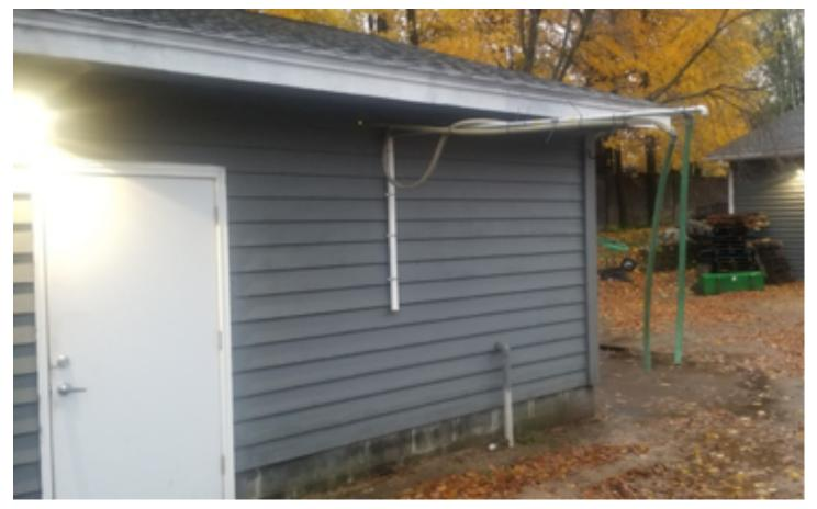
The Solubilizer 1000 was plumbed directly using washing machine hook ups. We added an extra water spigot for helping to mix and for rinsing. We then plumbed the discharge from the washing machine pump up and out for easy loading.
