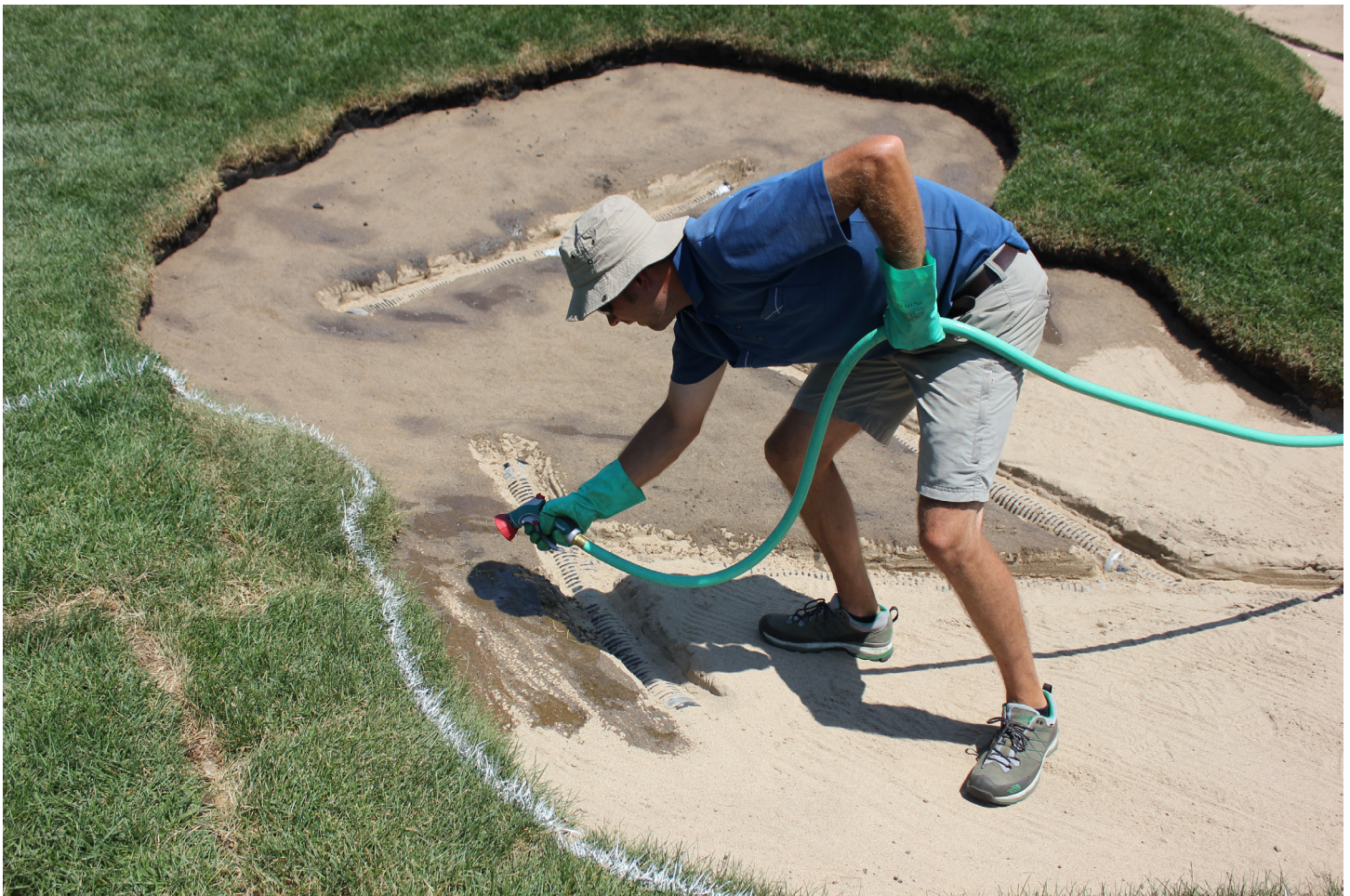
Klingstone is applied to stabilize the bunker base, prevent contamination and enhance drainage.
