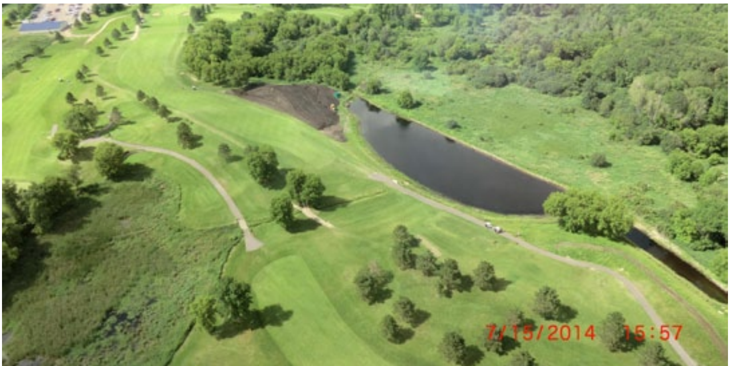
The newly created containment pond on Oneka Ridge Golf Course captures phosphorous laden water from urban and agricultural runoff.
