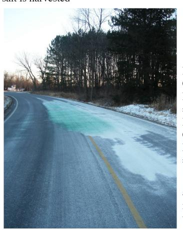
to achieve good results. Liquid chlorides are hygroscopic which means that they 'collect' moisture. Their molecules seek out water and bind with H2O molecules. The result is a liquid solution on the surface with a much lower freezing point. The benefit is that snow or ice won't adhere to pavement. It creates a non-stick
