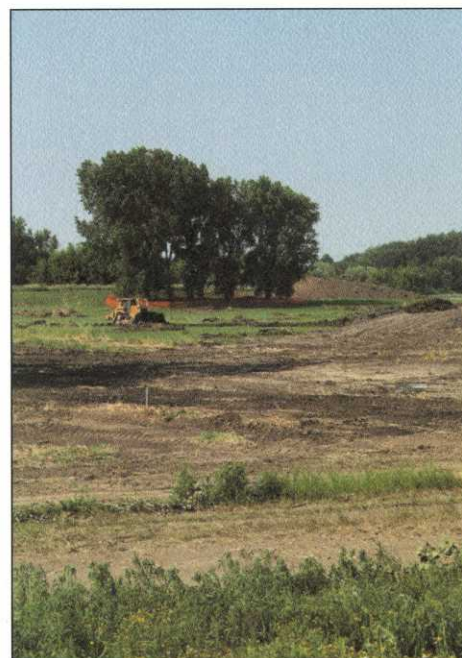
Wayzata CC's renovation begins on the range.
