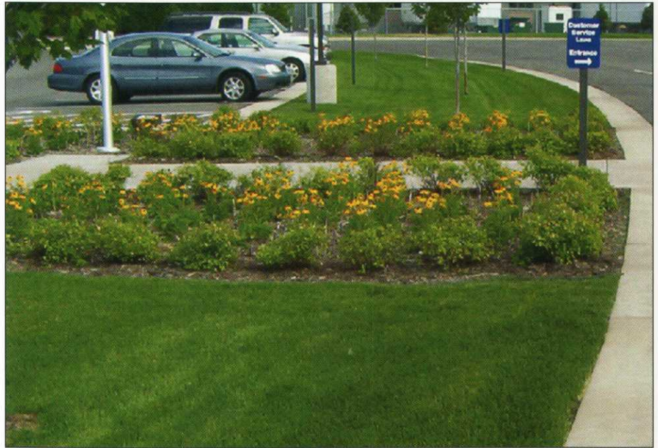
Lawn and landscaping used for infiltrate and filter stormwater runoff from adjacent hard surfaces.
